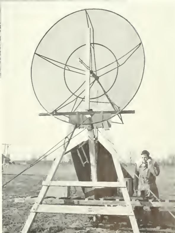
ENGINEER TUNES SLOT-TYPE ANTENNA BEFORE IT IS LIFTED TO TOP OF 210-FOOT TOWER OF BRIDGEPORT STATION.
