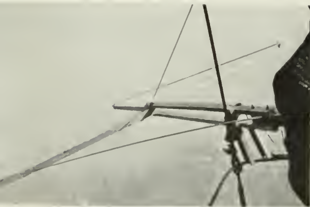
1931—THIS "DIAMOND" ANTENNA WAS INSTALLED ON THE 105TH FLOOR PARAPET OF THE EMPIRE STATE BUILDING.
