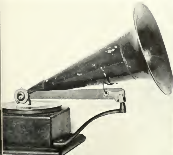
THE BERLINER GRAMAPHONE, PATENTED IN 1887, FEATURED A FLAT DISC AND A HORN, IN CONTRAST TO THE CYLINDRICAL RECORDS THEN IN COMMON USE.
